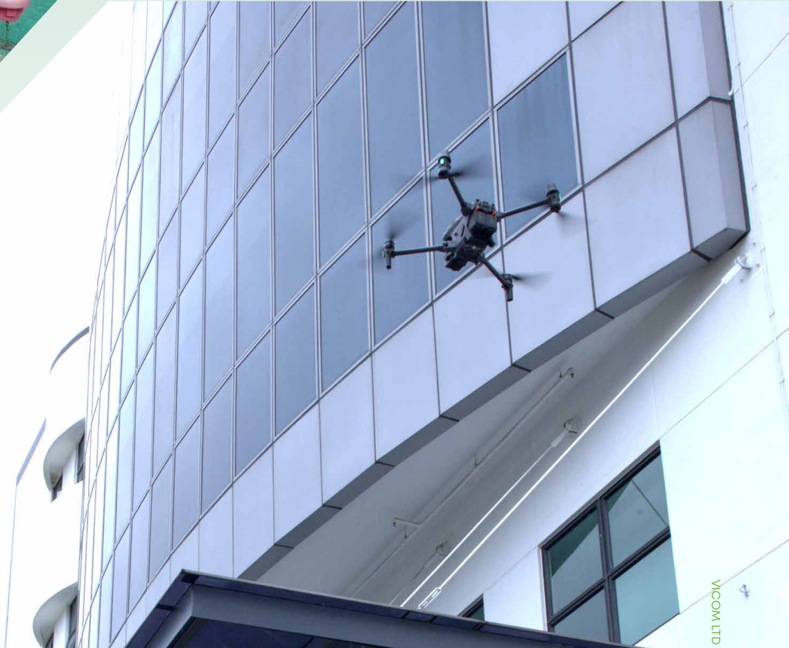
Facade inspection using drone technology to increase productivity.
